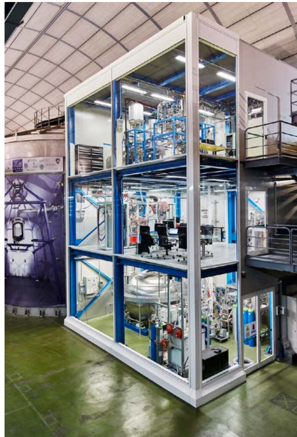
XENON1T underground infrastructure includes the water tank and cryostat, electronics, gas storage, and purification.
